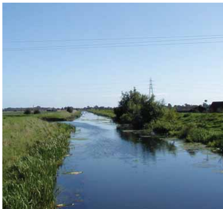
River Steeping at Thorpe Culvert, within the LDMU
