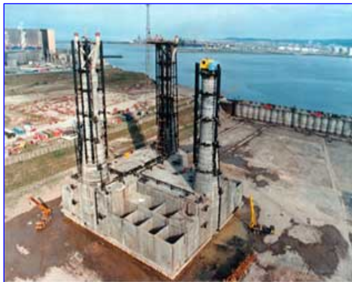
Figure 2.2 Dry Dock at Able UK 1
