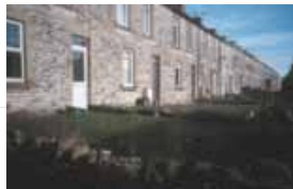
Alexandra Terrace, Ham Lane, built of squared coursed rock faced white lias rubble with oolitic limestone dressings, terrace steps down contour to east, double Roman clay tiles with decorated serrated clay ridge with low boundary walls of white lias stone with cock and hen capping
