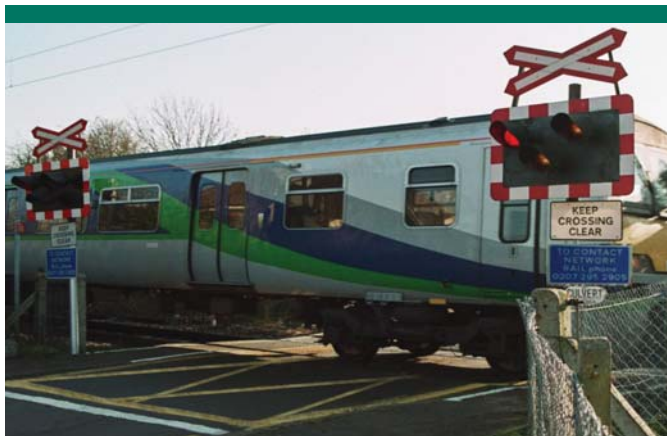
At this un-gated crossing the carriageway is less than 5.0 metres in width and the centre lines have been omitted. See Traffic Signs Manual, Chapter 5 9 , Railway Level Crossings.
