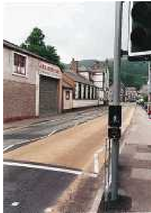
Alternative nearside signal arrangement showing pedestrian green signal and a pushbutton
