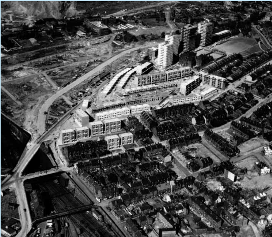
Aerial Photograph of the Woodside site in 1961
