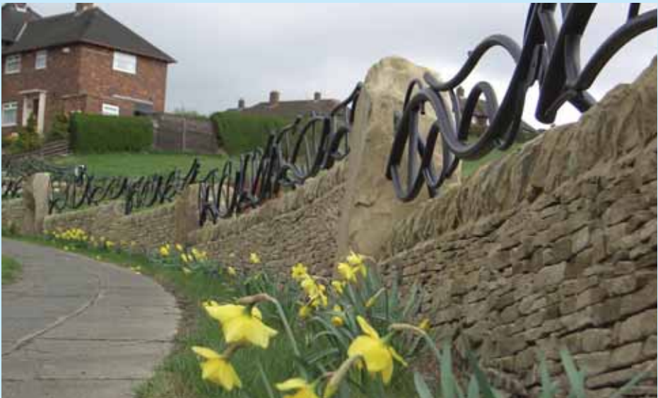
Railing Detail from Manor Fields Park, Designer Chris Campbell
