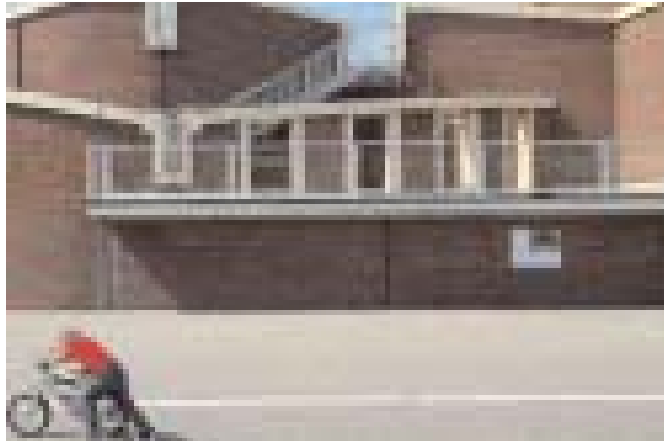
The red brick building at Eastbourne houses the control room and a sludge processing plant
