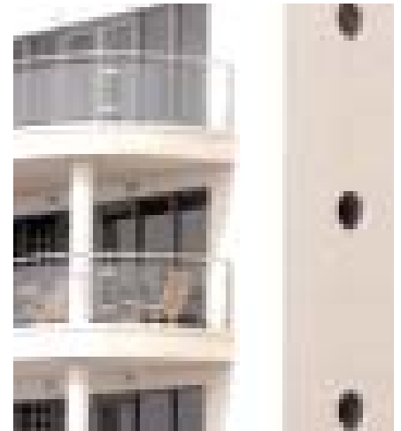
Detail of the apartment block showing glass-fronted balconies
