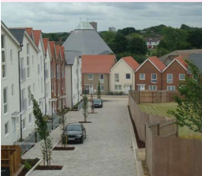
The first houses, designed by Fraser Brown McKenna Architects, are nearing completion
