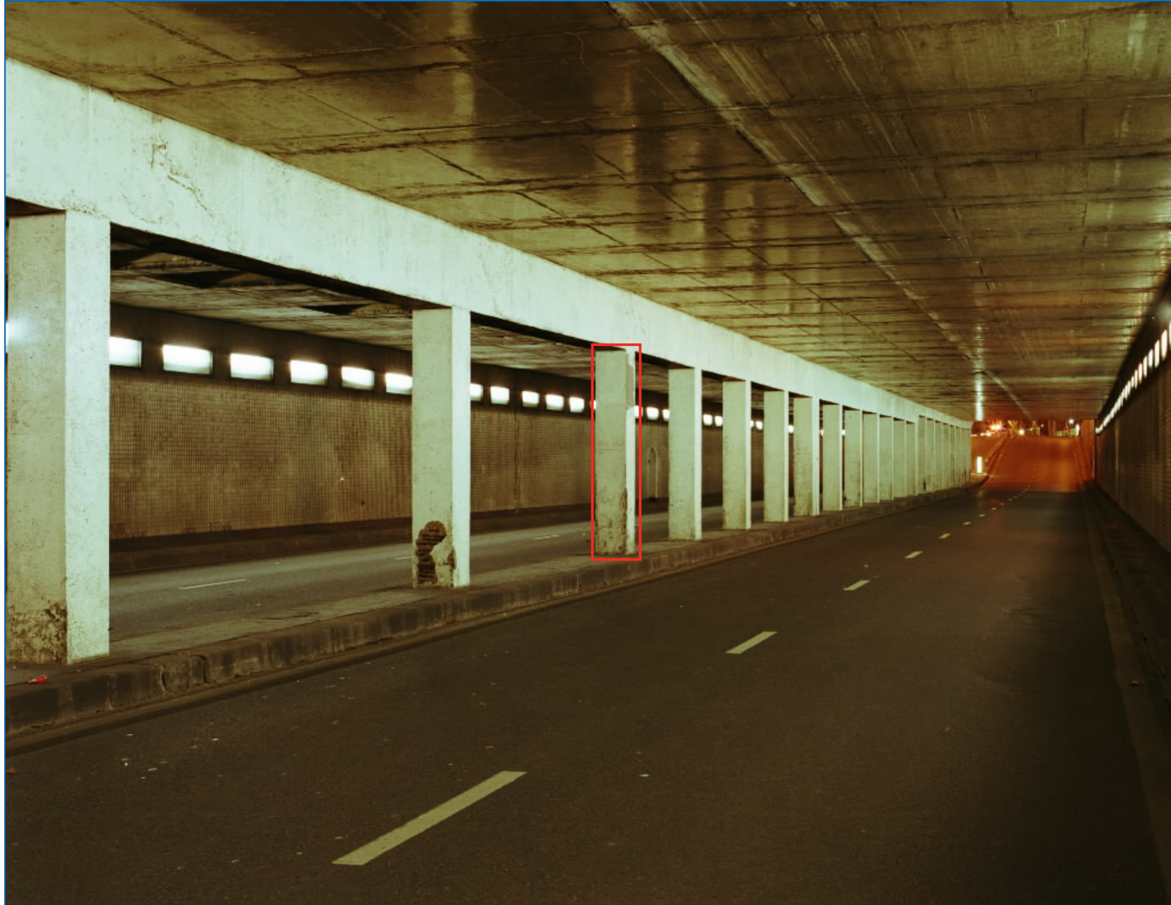
Alma underpass, 13th pillar highlighted
