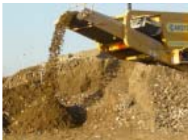
Figure 7.2 Screening of excavated material to be reused as sub-base.
