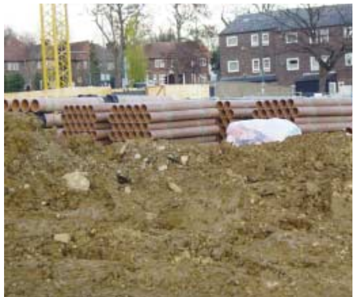
Soil as a platform for construction
