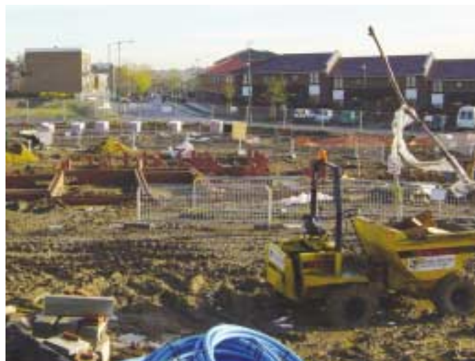
Construction of new housing on brown field site
