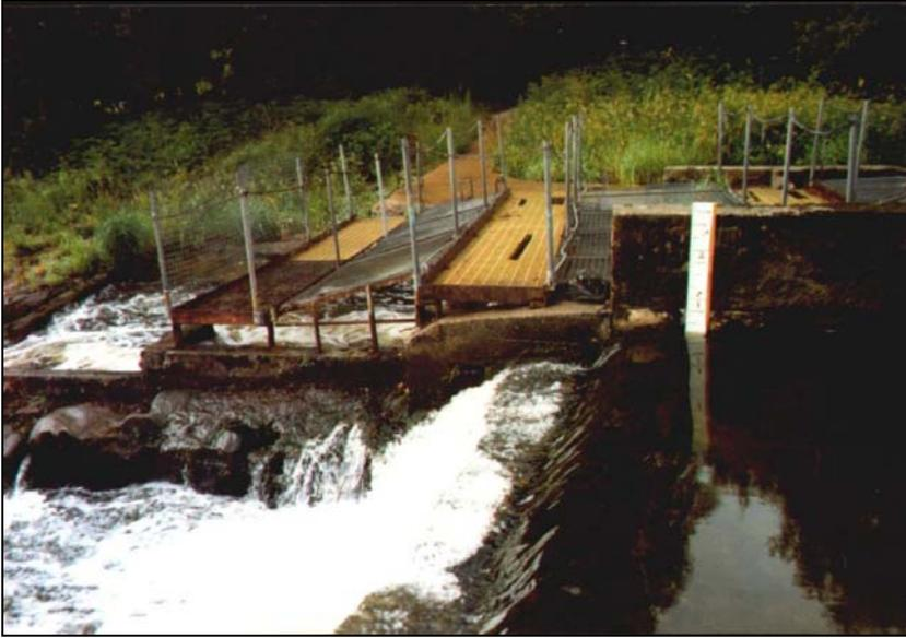
**Figure 6. Gunnislake Weir on the River Tamar with the associated fish pass and trap (Cornish side).**
