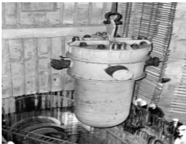
Civil PWR RPV being lifted.
