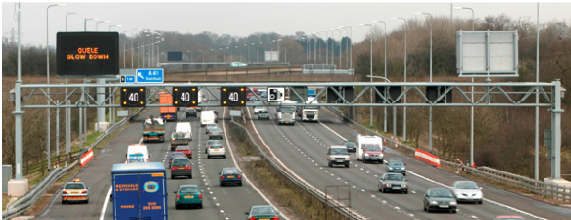
Figure 3 Lightweight Gantry on the M42 (Source HA)
