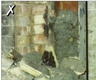
Limpet/sprayed asbestos
