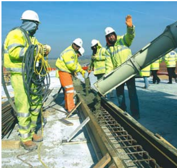
Pouring concrete on A249 Sheppey Crossing
