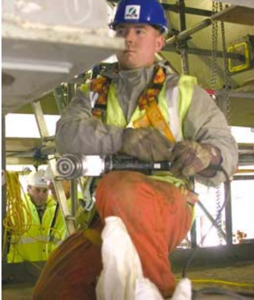
Using skills to extend life of heavily trafficked M6 Thelwall Viaduct
