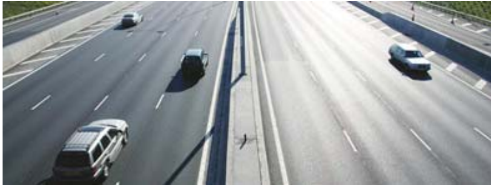
M25 J12-15 widening
