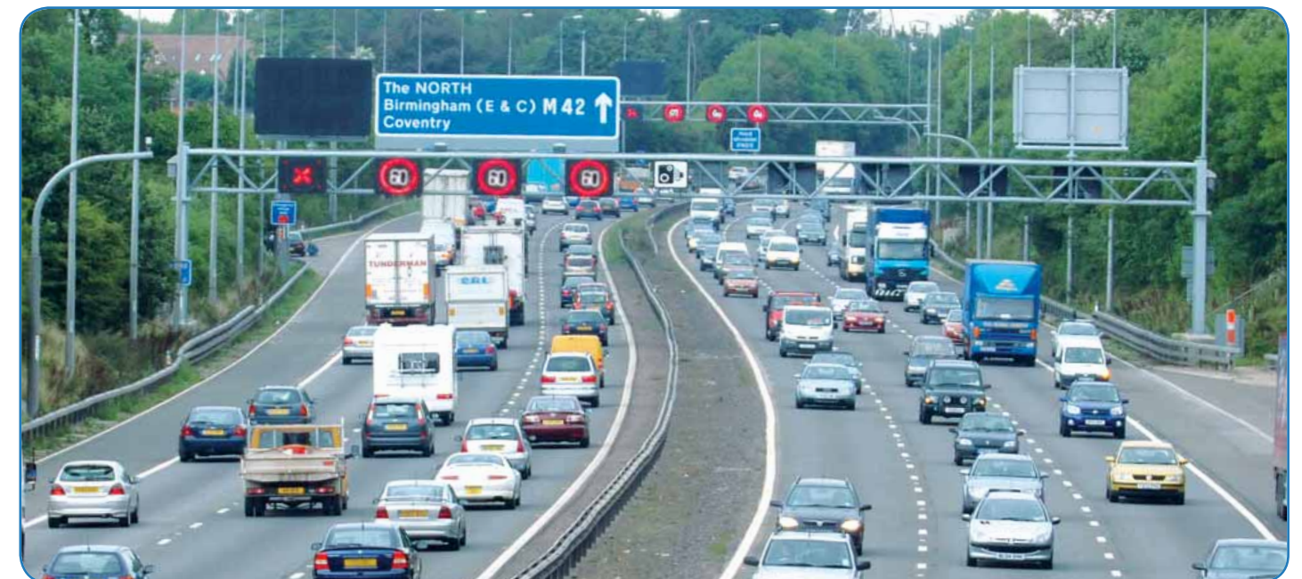
Figure 4. Dynamic hard shoulder running cross section
