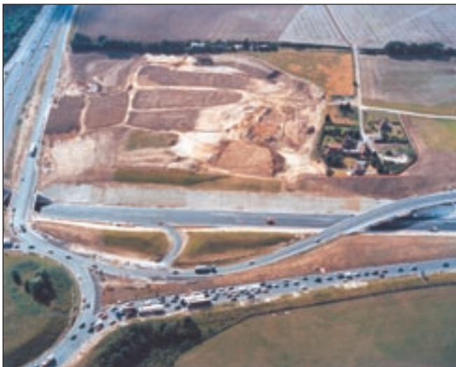
A34 North of Underpass & Radnall
