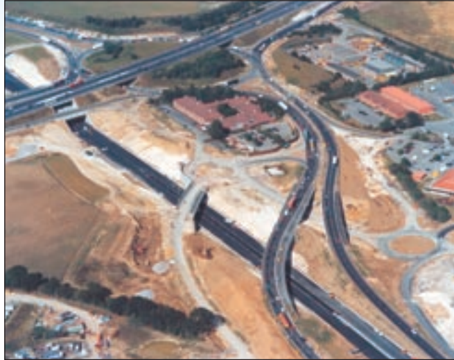
A34 Underpass looking north east
