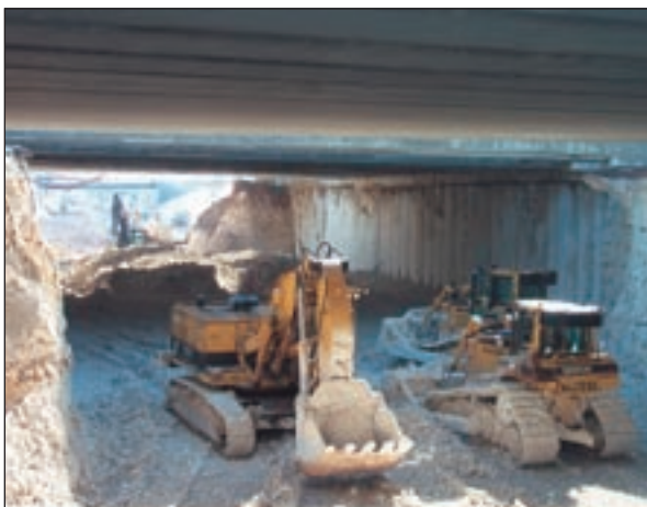
Excavating beneath the new bridge deck
