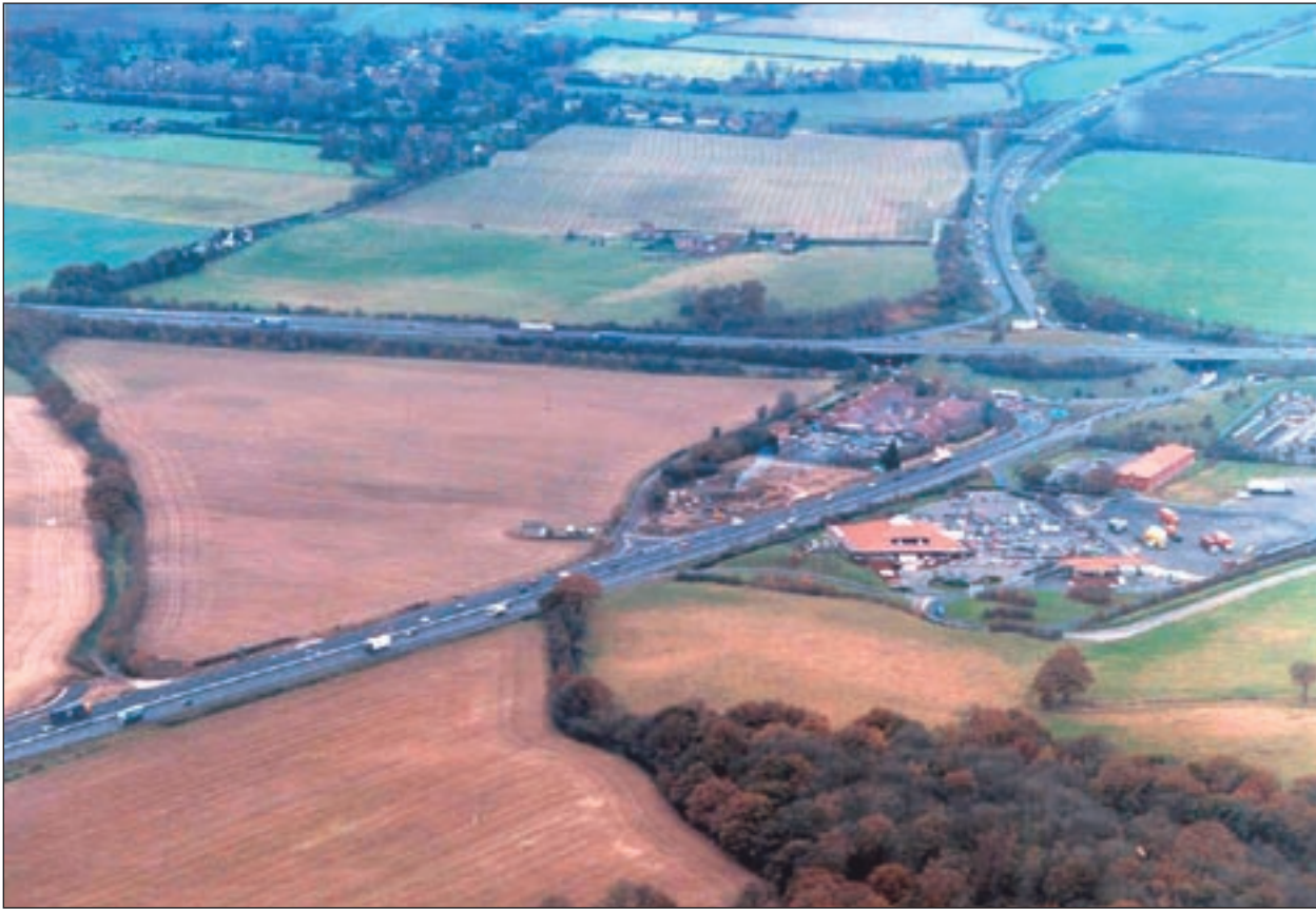
Before Works Commenced
