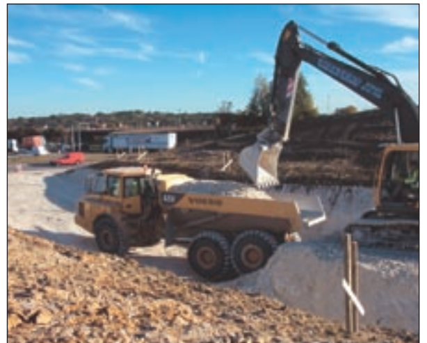
Excavation of the Police Observation Platform
