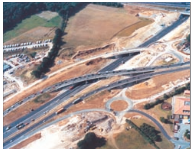
Junction 13 slip roads south of underpass
