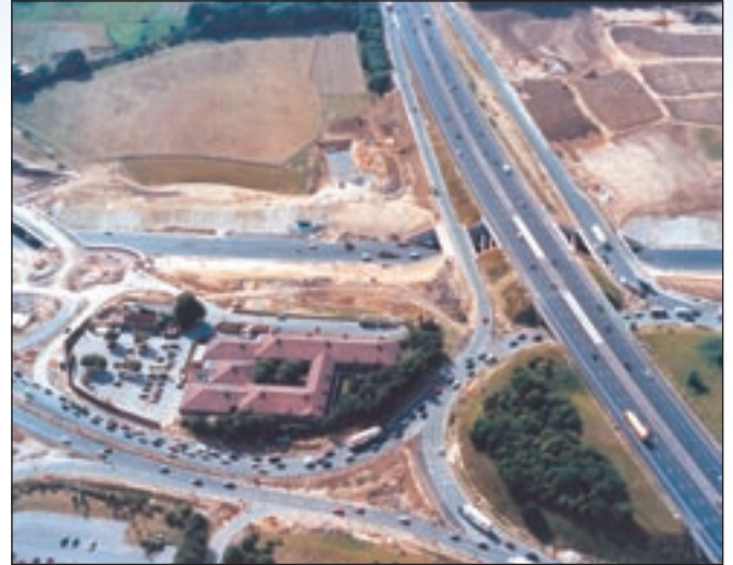
A34 Underpass looking west on M4
