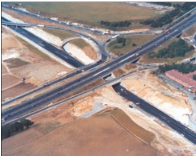
A34 Underpass looking north east
