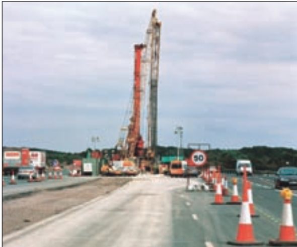
Works in Central Reservation of M4
