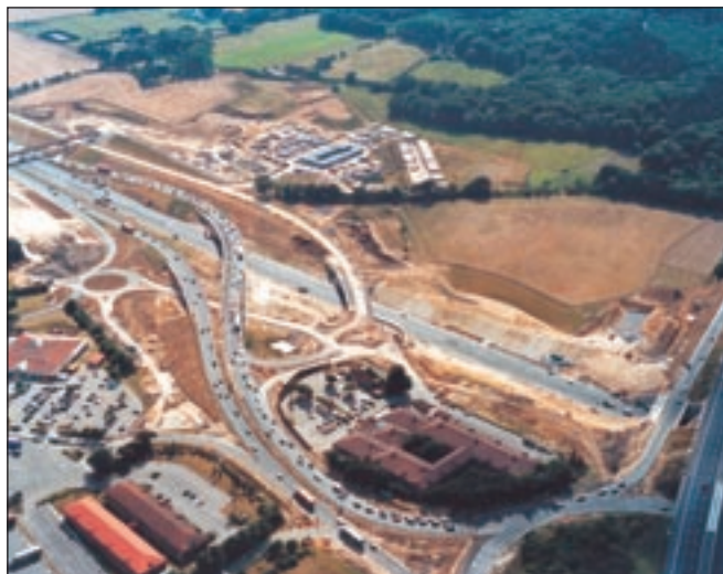
A34 Underpass looking south west
