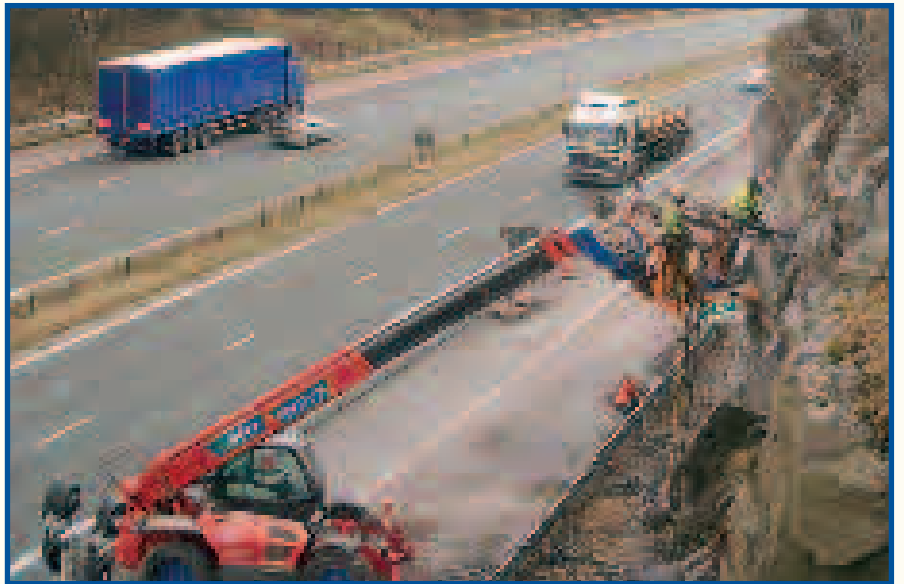
Work on the M6 rock face
