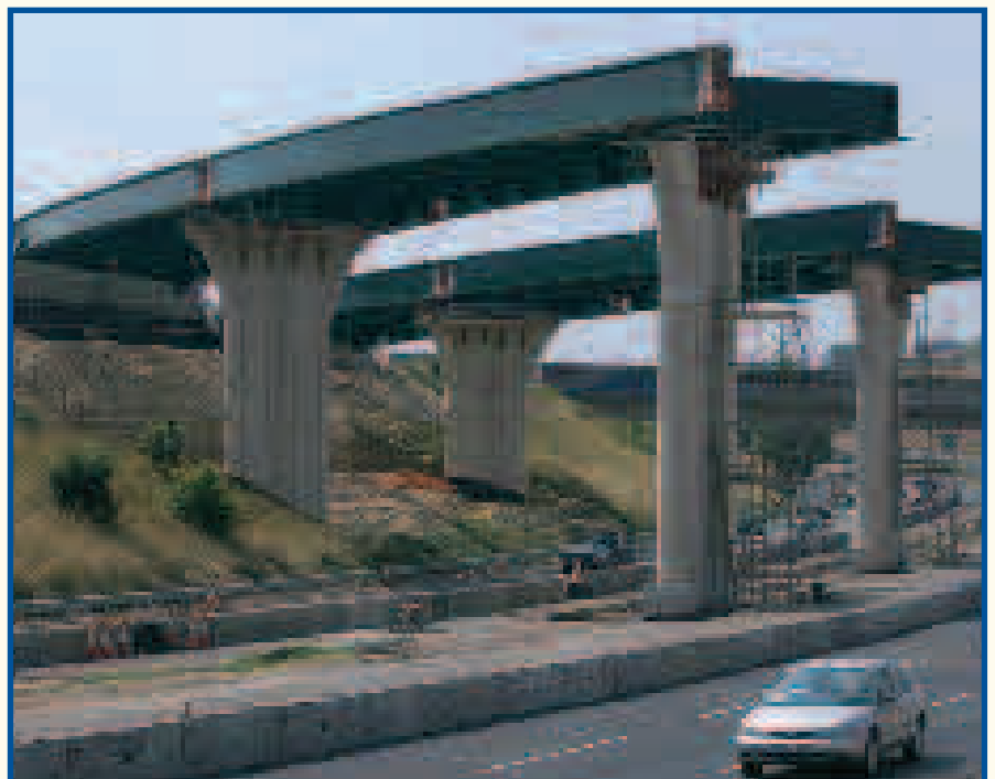
Ferrybridge Motorway interchange, M62
