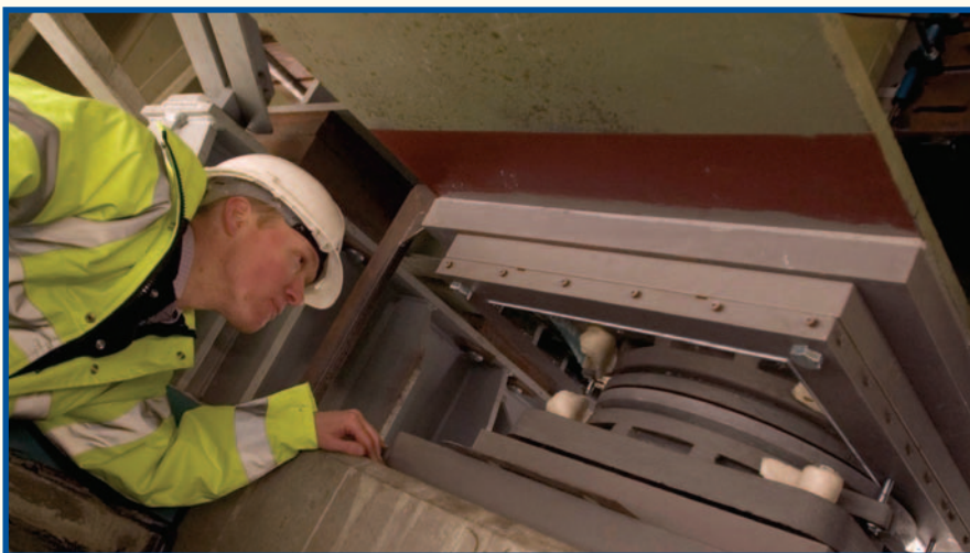
M6 Thelwall viaduct under major repair
