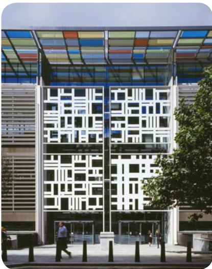
Coloured glass canopy and brise-soleil screen by Liam Gillick at main entrance of the new Home Office building, London
