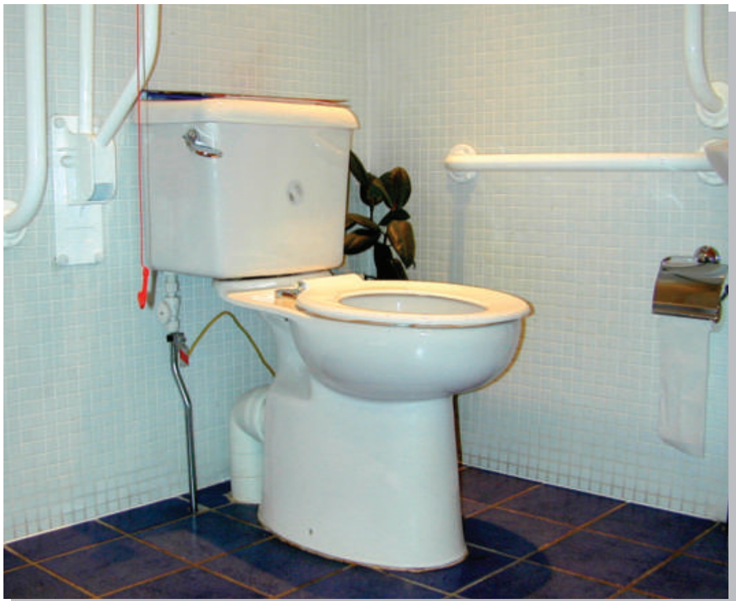
An example of an accessible toilet.
