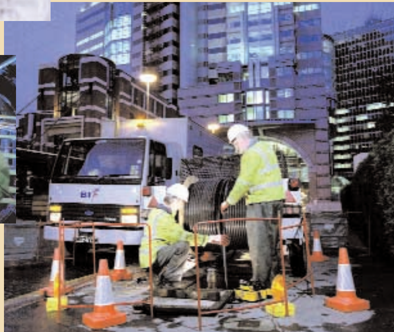
BT cable laying in City of London.
