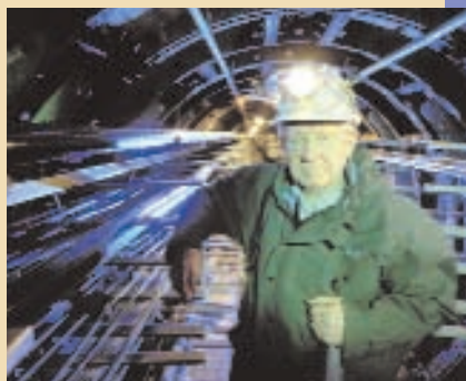
BT engineer repairing and maintaining underground cables.
