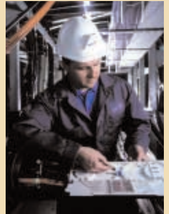
Engineer working on underground cables.
