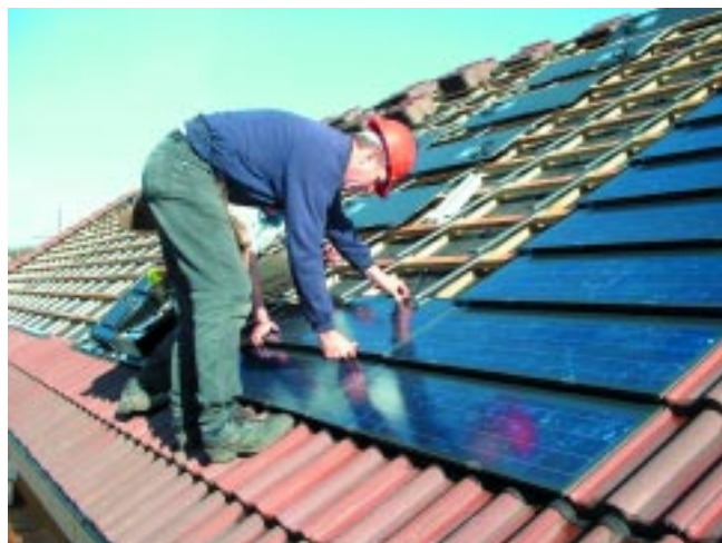
The tiles being installed (photo CDS)
