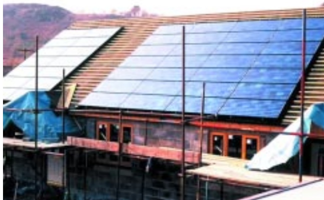
Installation in progress (photo Dulas)
