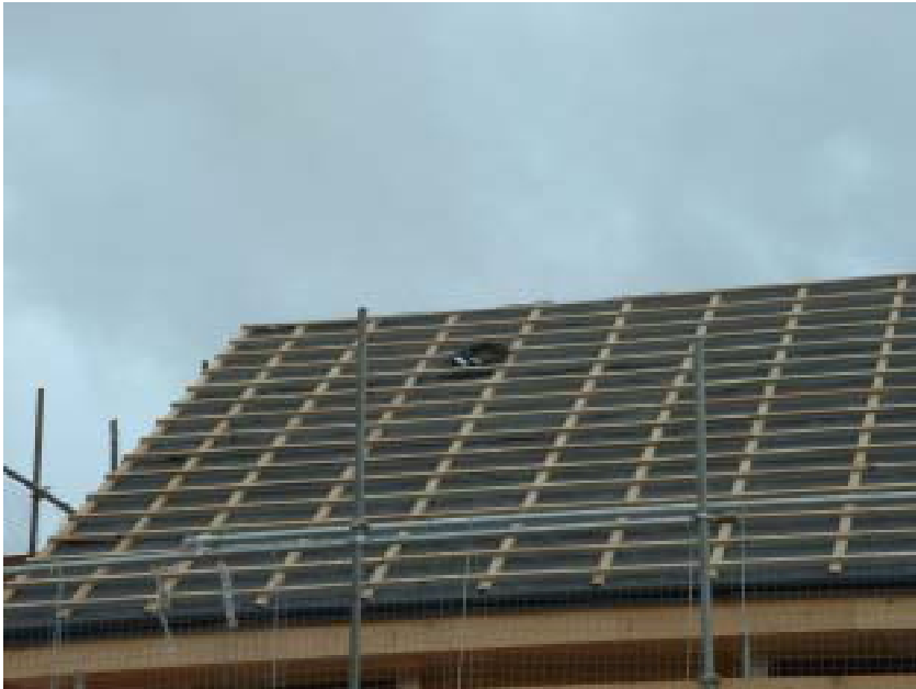
Fig. 22: Counter battens (verticals) installed correctly for cooling, beneath battens
