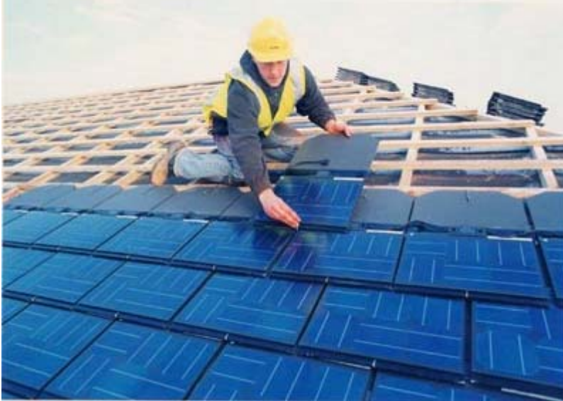
Fig. 27: Atlantic Solar Sun Slates being installed (Solar Century).
