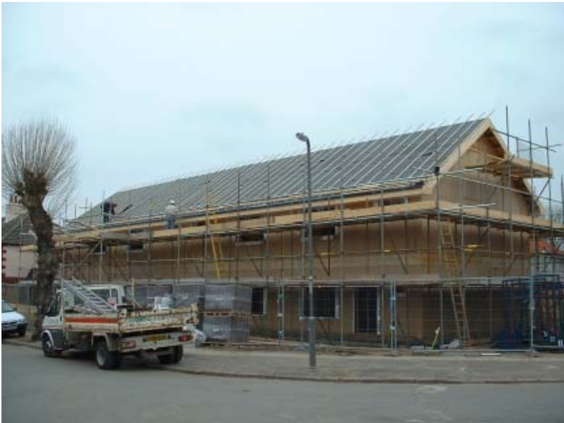
Fig.4: The new build block on the existing Pinehurst estate (BRE).
