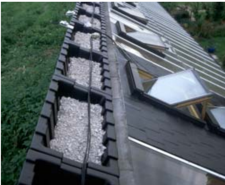
Fig. 31: Consoles ready for panel installation.
