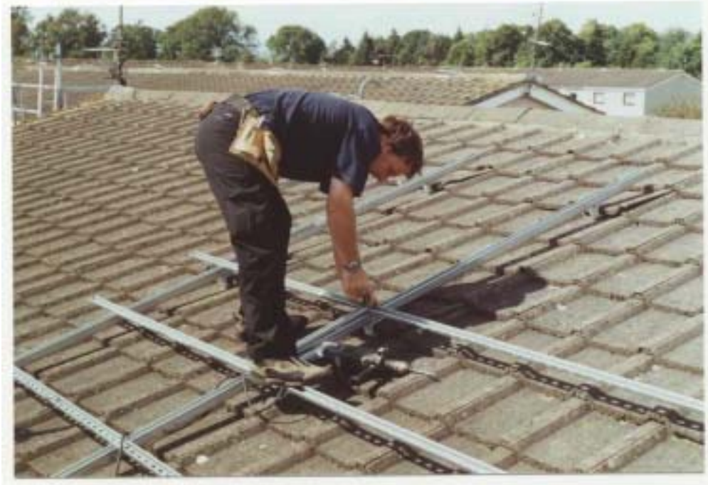
Fig. 30: Installing the Unistrut frame to the roof hooks (BRE).
