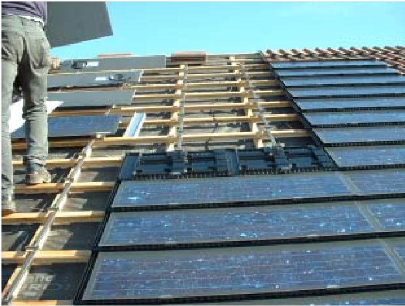
Fig. 23: Plastic trays for weatherproofing with modules fitted on top
