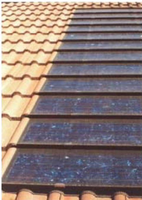
Fig. 24: The finished installation at Pinehurst (BRE).
