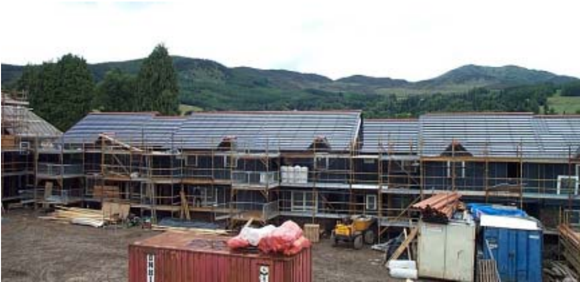
Fig. 11: The Pitlochry development (Perthshire HA).
