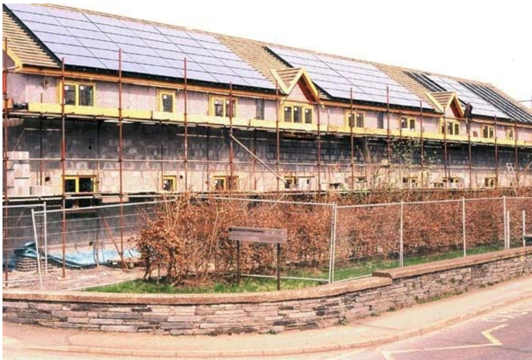
Fig.1: The Machynlleth development under construction. (Dulas)
