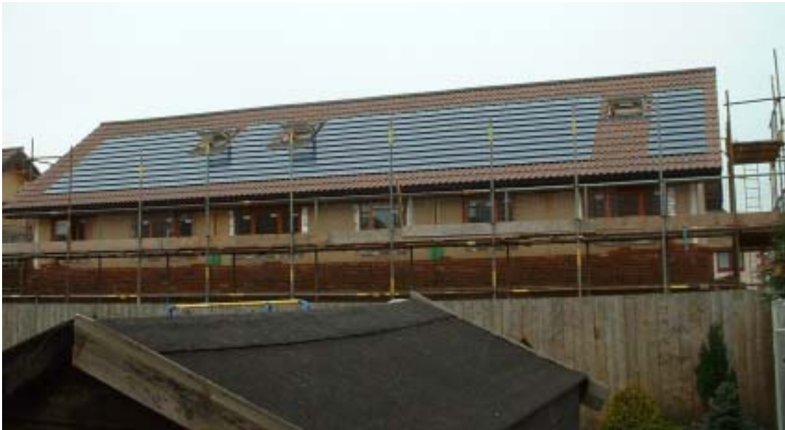
Fig. 6: Integration of roof windows at Pinehurst (BRE).
