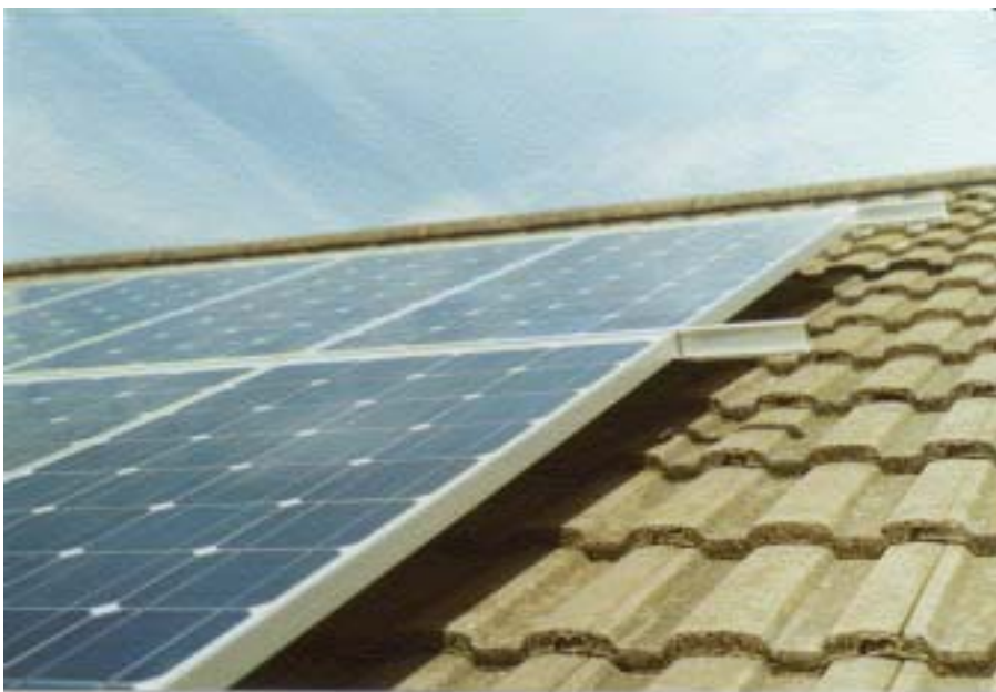
Fig. 28: Detail photograph showing modules and Alutec frame (BRE).
