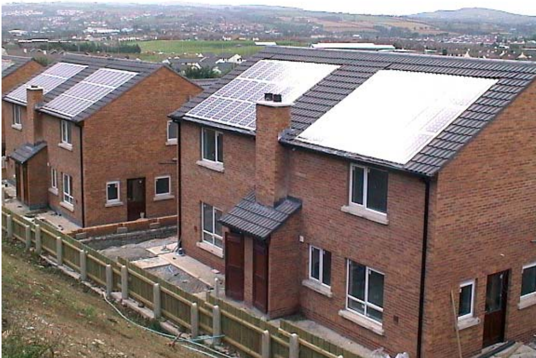
Fig. 19: PV arrays are integrated into the south-facing roof using the PV systems "RIS" system.
