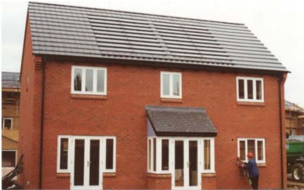
Fig.7: Pfleiderer roof integrated PV at Broughton Leys (BRE).
