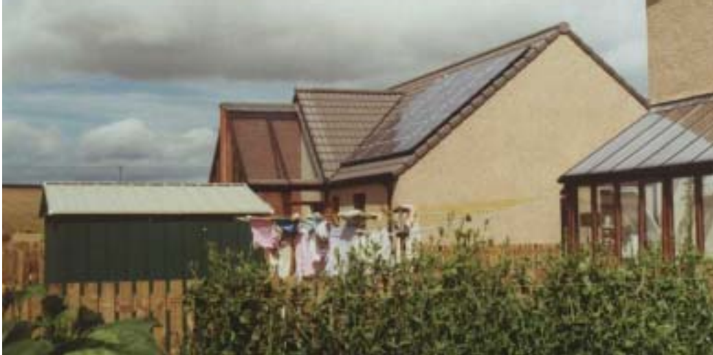
Fig.16: Retrofit PV arrays at newer houses in Lawfield, Ayton (BRE).
