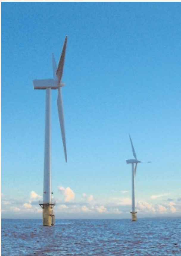
Blyth offshore wind farm
