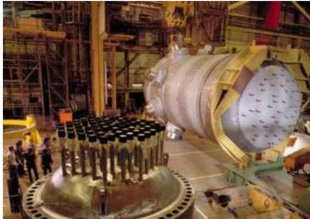
Figure 8 – Reactor Pressure Vessel (RPV) and integrated head manufacture (courtesy of AREVA NP).
