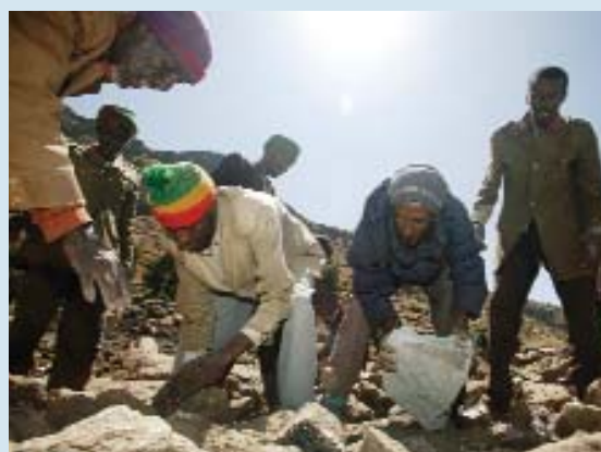
Road building in Mekelet Village, Central Highlands, Ethiopia
