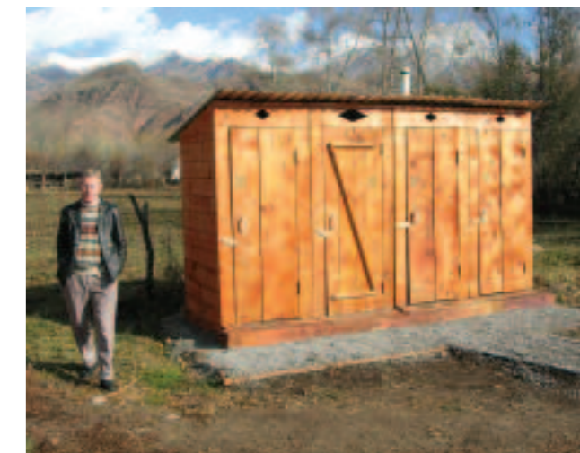
New latrines in Kyrgyzstan provide privacy, convenience and improved standards of hygiene for local people. David Sutherland
