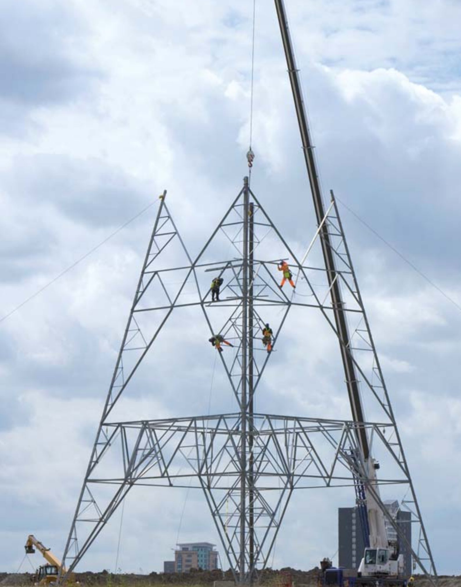
De-construction of electricity pylons on the Olympic Park site
