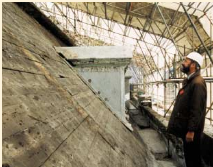
Roof of No.4 Store, Morice Yard in course of repair
