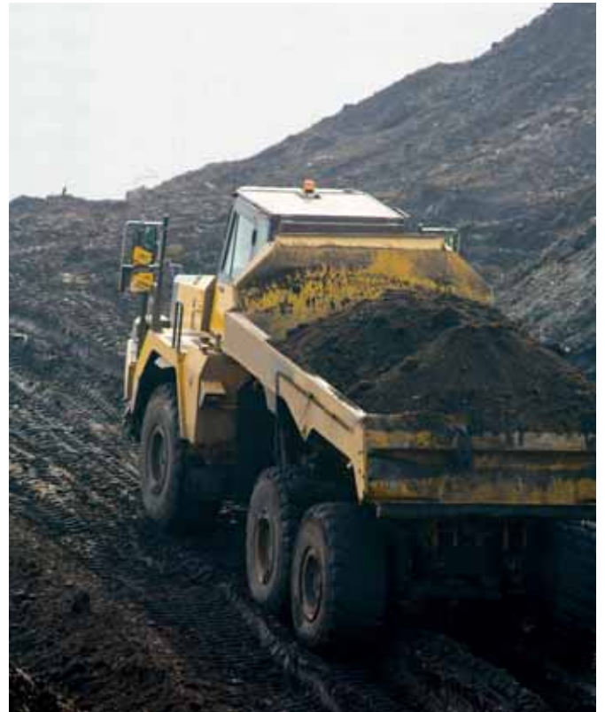
Clearing the rubble from the Olympic Park ready for construction
