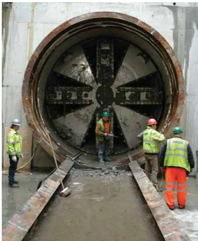
Construction workers at the underground powerline tunnelling for the Olympic Park
