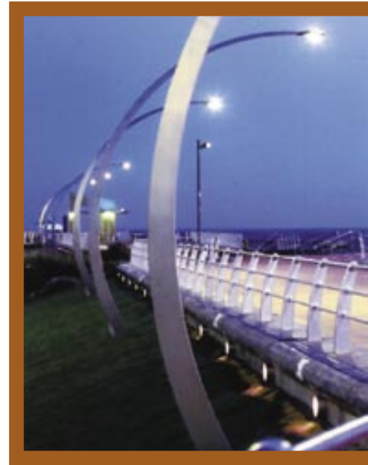
Delivering on the Fylde Coast: part of the £80 million remodelling of the promenade in Blackpool
