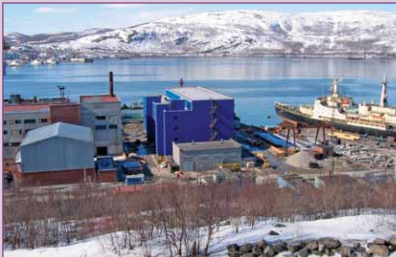
Building 5 (centre) interim SNF store at Atomflot, Murmansk, NW Russia
