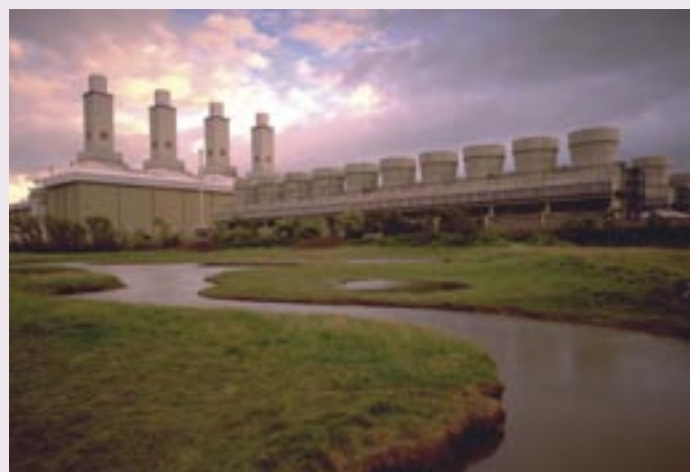
Connah's Quay Power Station and Gas Treatment Plant (courtesy of Powergen).
