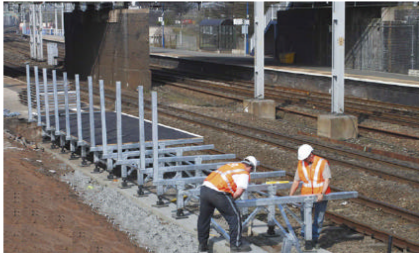
Installing a steel modular platform at Lichfield station
