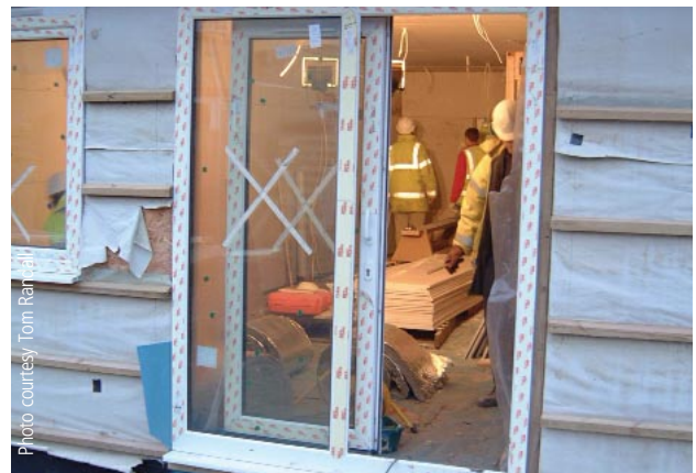
▲ Habitat for Humanity work in progress
