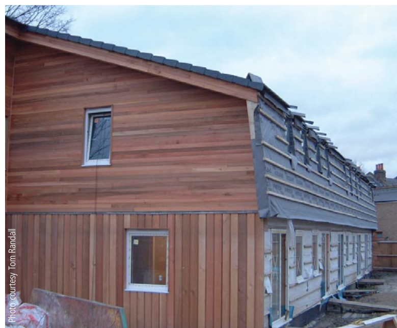
▲ Habitat for Humanity wooden cladding
